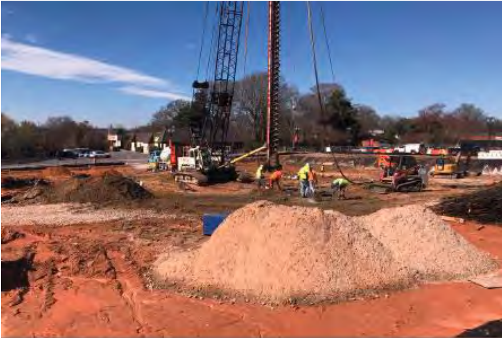
Augercast Pile Install
