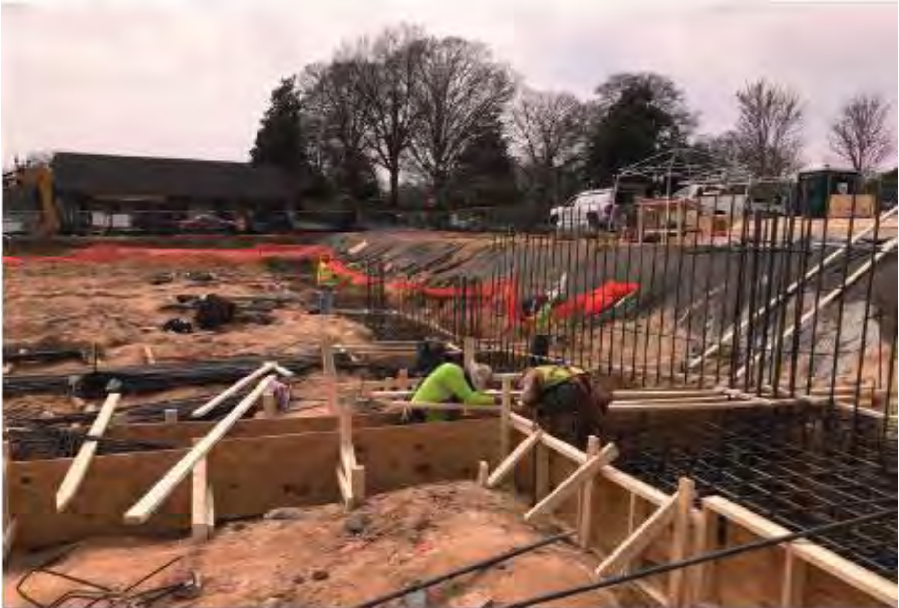
Shallow Foundations & Retaining Wall Rebar
