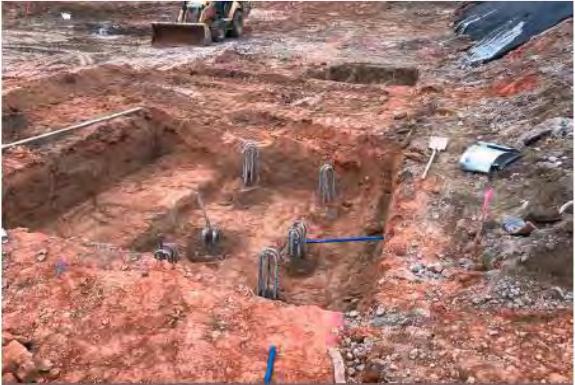
Pile Cap Excavation
