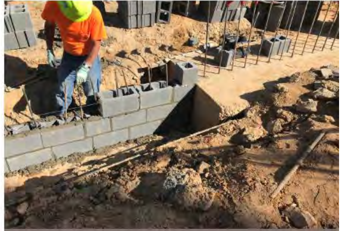
Masonry Retaining Wall Installation
