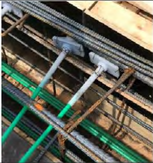
Photo 9 Tendon anchorages at CLL-8
