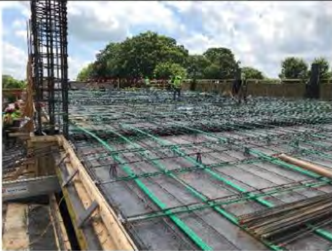
Photo 11 Tendon layout (looking west)
