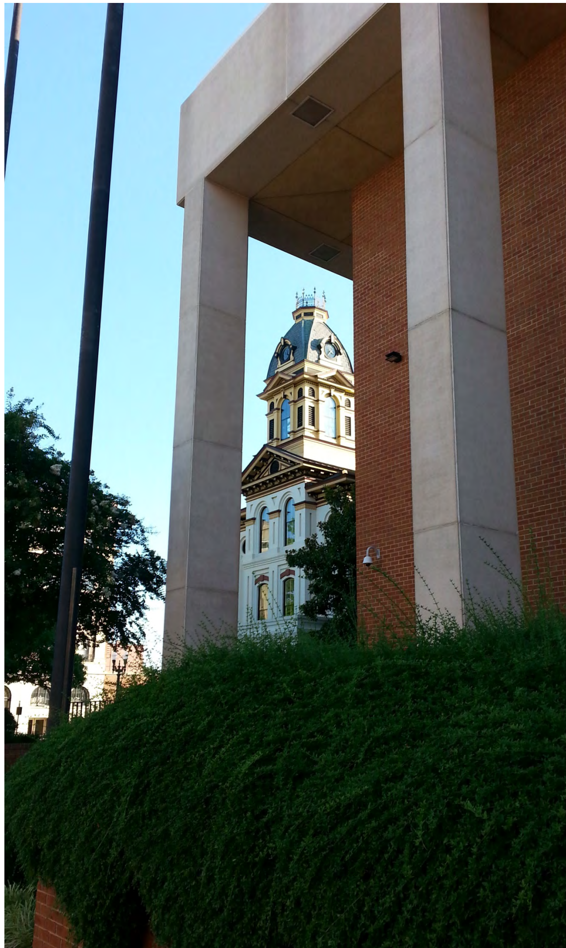
Existing View of Historic Courthouse at Corner
