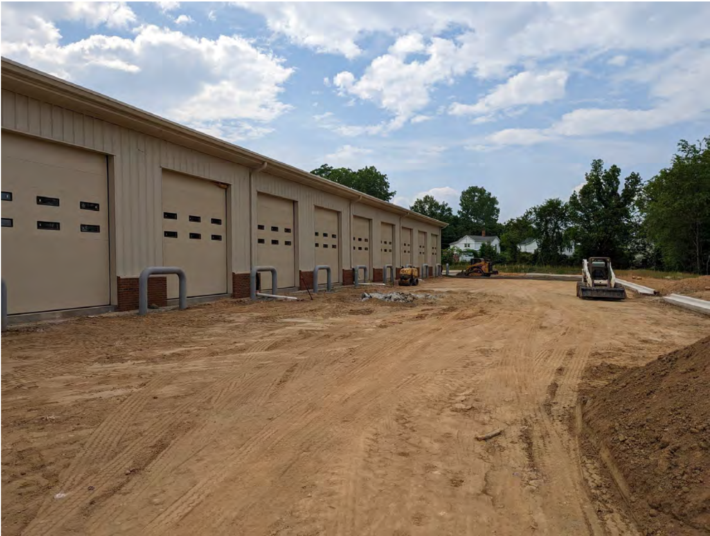
Back side of the warehouse
