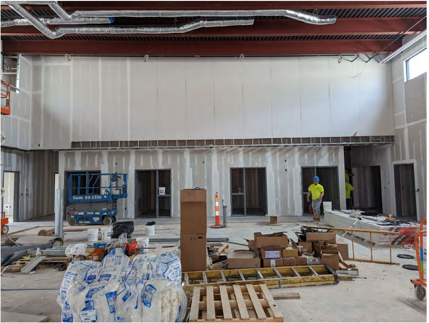
Open office space area in the ITS building
