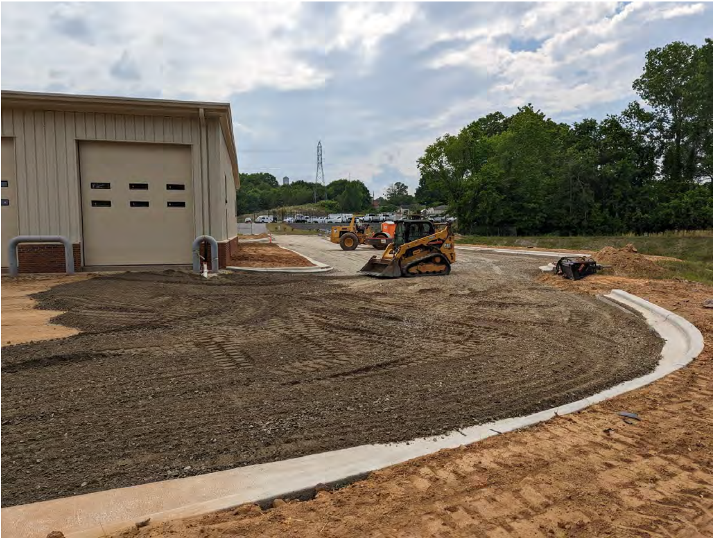
Back of warehouse working on putting down gravel in parking lot
