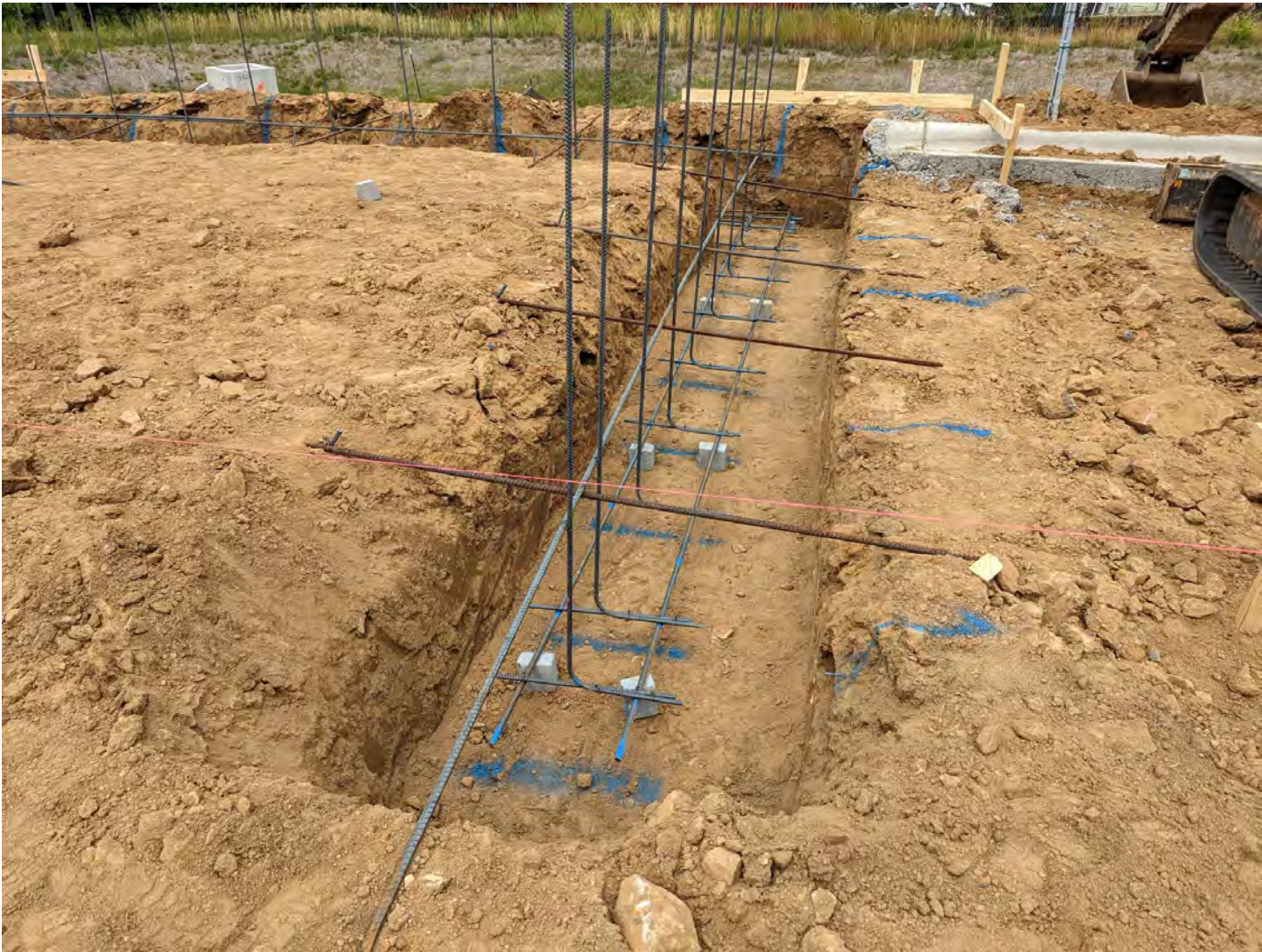
Dumpster enclosure footings
