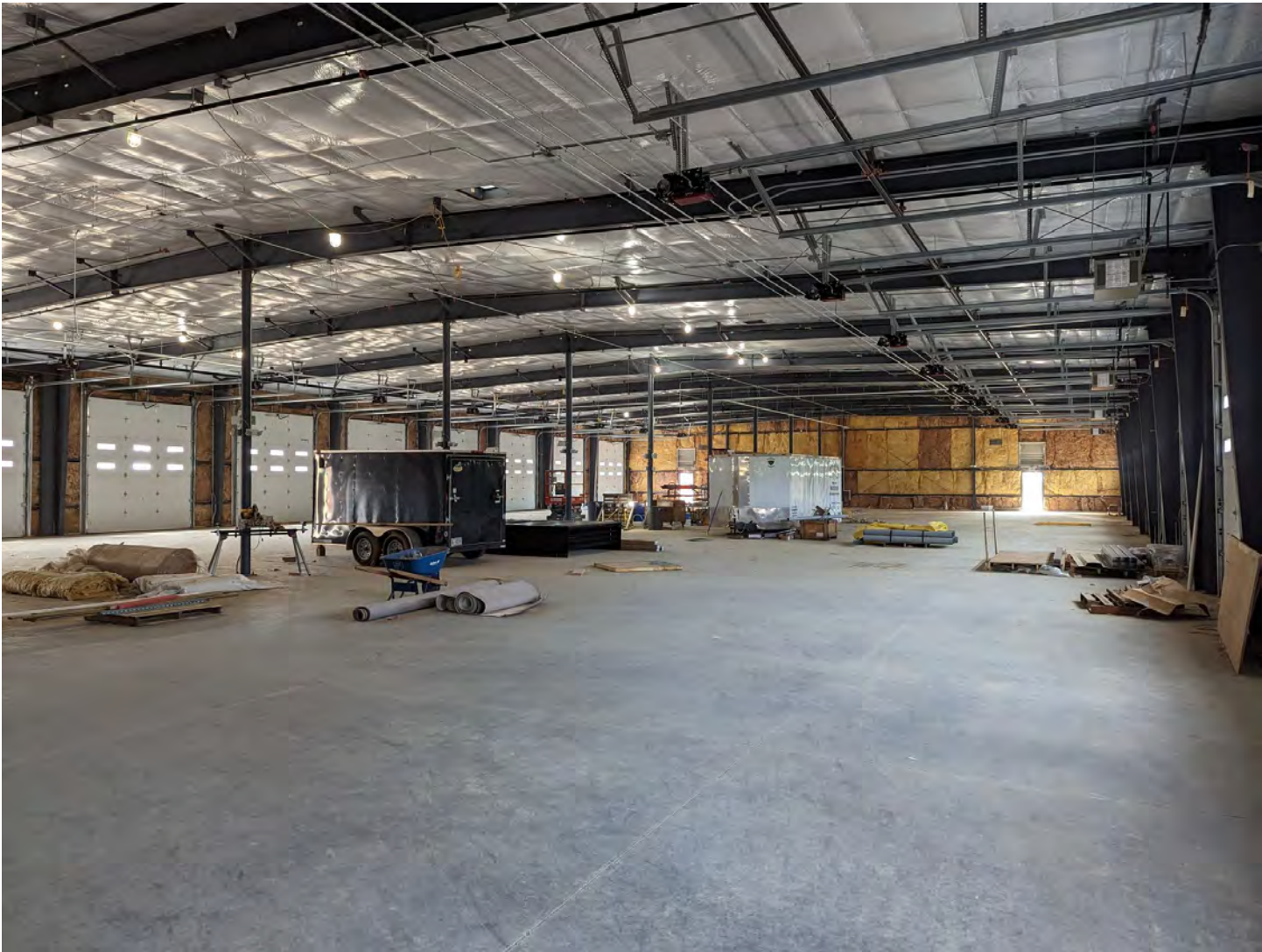
Inside view of the warehouse space
