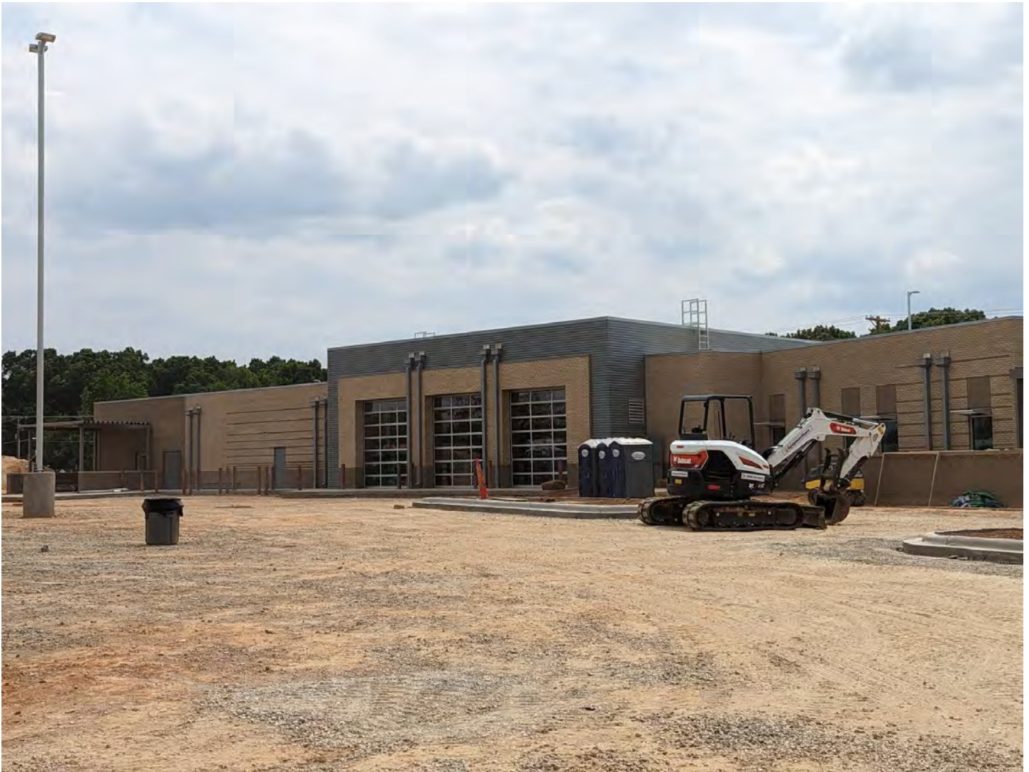
Back side of the building looking at the ambulance bays
