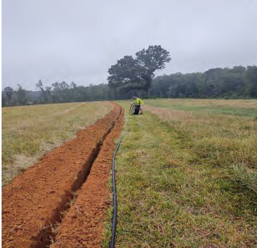
Trenched water line for livestock drinker
