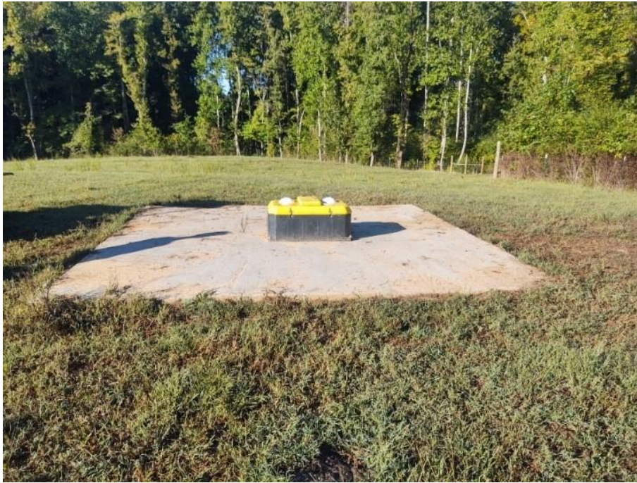
Heavy use area with installed drinker
