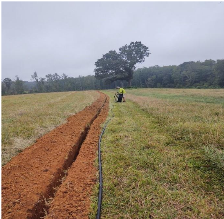
Trenched water line for livestock drinker
