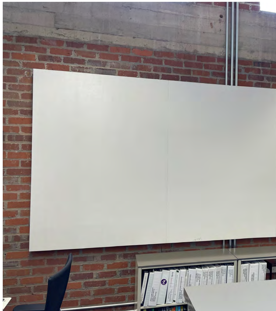
Strategy #1 Exposed Acoustic Wall Panels (If mounted high enough to be out of reach for users)
