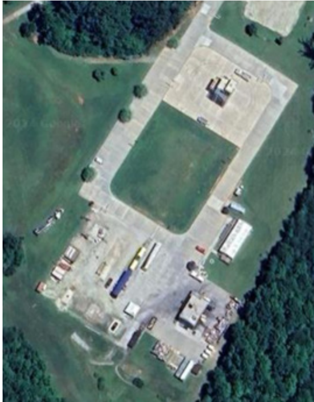
RCCC Fire Training Area Overview
